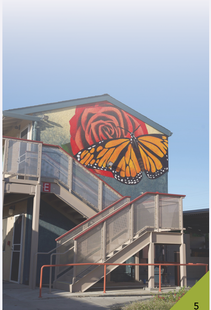
Idaho Apartments, El Cerrito
